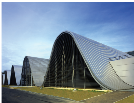
Research Center, Gif sur Yvette - France Architects: CEA / Vasconi Associés © Philippe Ruault
