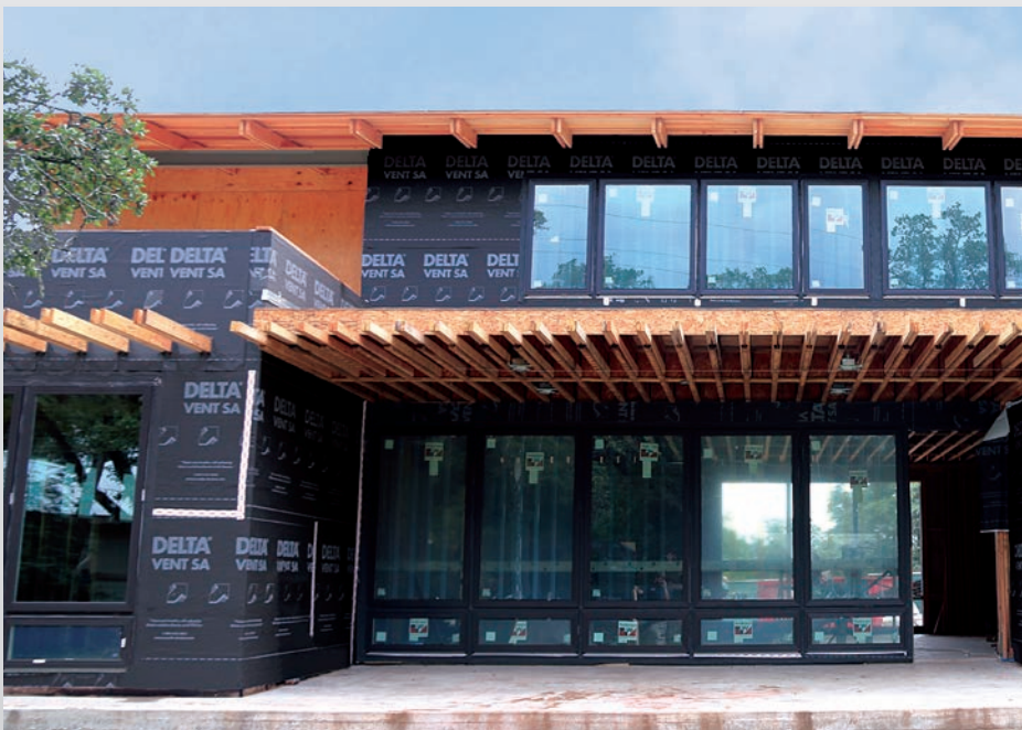
Air barrier application in residential construction
