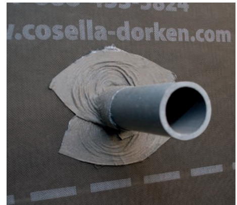
Air barrier continuity at penetrations
